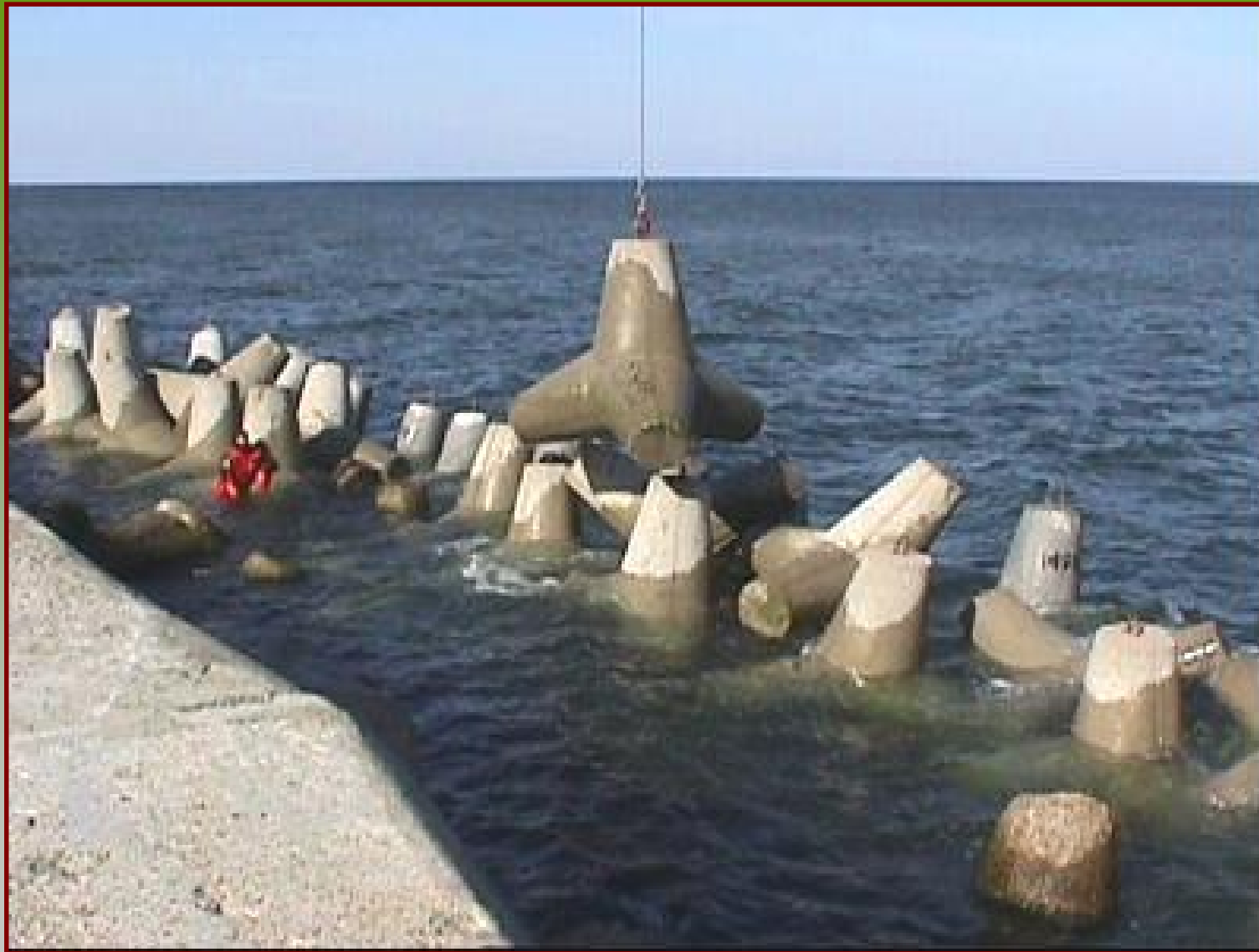
Reconstruction of armour at Wladyslawowo harbour breakwater in September 2003
