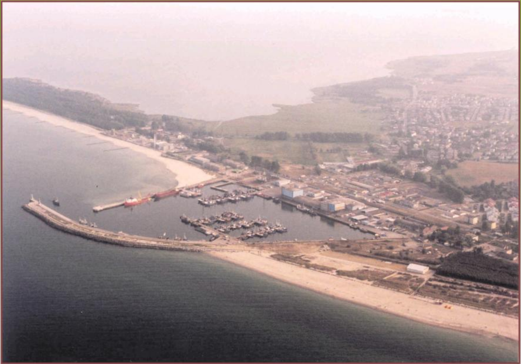
Władysławowo harbour: accretion on west side (bottom), lee side protected by groins and beach fills (top left hand side)
